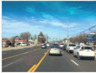
Continuous Center Turn Lane
